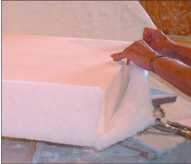
When fiber is applied to foam, fast tack time with a longer open time is necessary to allow the fiber to be worked into place.
